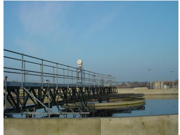
Partech offer a selection of sensors for use in conjunction with our range of Sludge Blanket monitoring instruments. All the sensors use infrared attenuation as their operating principle, this makes them sufficiently sensitive for use on low density sludges (such as Final/Secondary Settlement) as well as the more usual sewage treatment applications.
